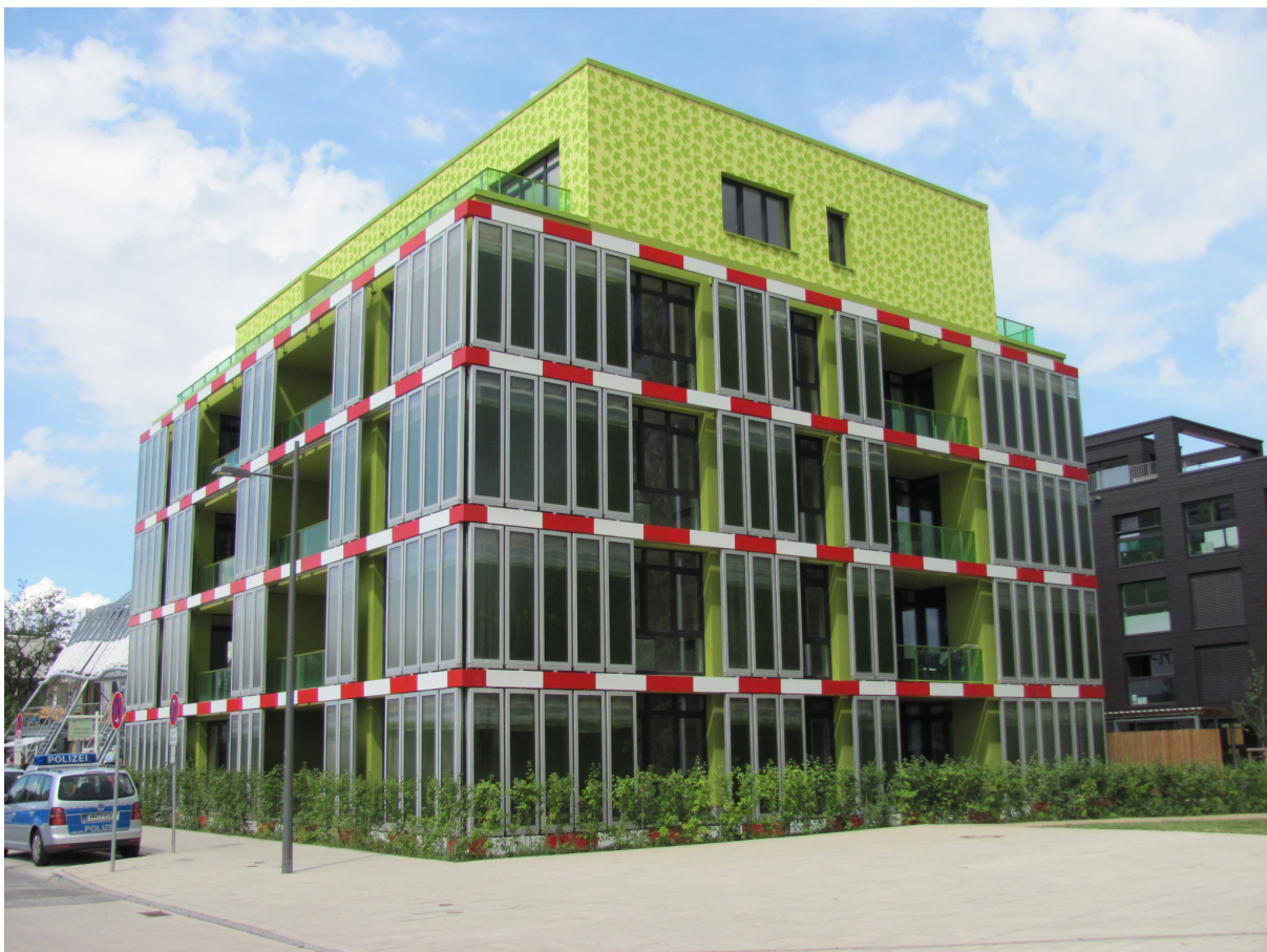
BIQ (Bio Intelligent Quotient), a building powered entirely by algae in Hamburg. Credit: NordNordWest (CC BY-SA 3.0) .
